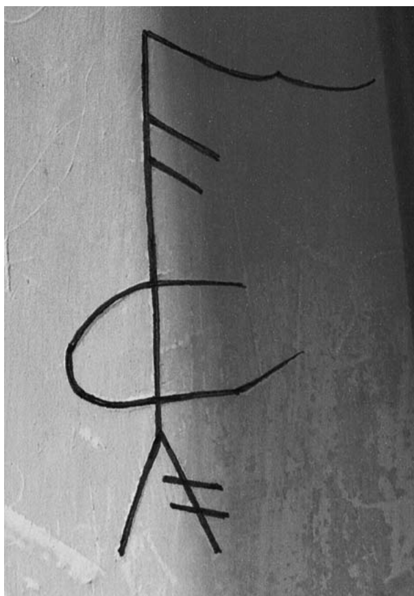
FIG. 99 – Tower arch, north side. Probable merchant’s mark inscribed in close proximity to the name of Johannes [John] Abthorp.
